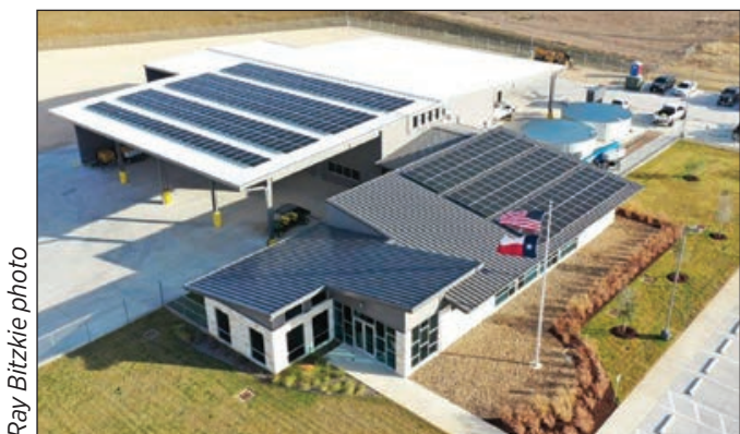
Bluebonnet's Maxwell service center has 292 solar panels that can offset about 70 percent of the facility's total annual energy consumption.
