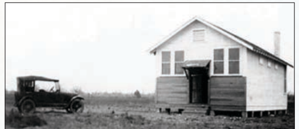
The Hopewell Rosenwald School in 1922. The building still stands at 690 State Highway 21. Source: Julius Rosenwald Fund Archives 1917-1948, Fisk University
