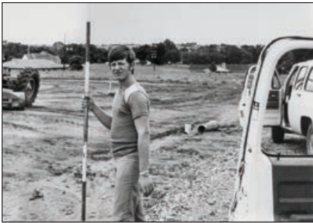
Above: Rodney Fritsche, a survey technician in the 1970s, helps determine the location of future power poles and lines.
