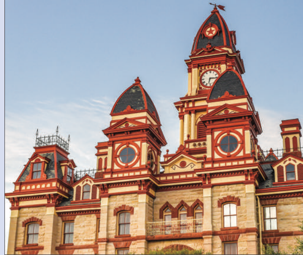
■ The Caldwell County Courthouse, at left, has appeared in movies and TV shows. Widely regarded as one of the finest courthouses in Central Texas, this ornate 1894 Second Empire-style structure dominates Lockhart's historic district. Unlike many courthouses in the area, the interior remains largely as it was when originally built, down to the elaborate hand-carved features on the wood staircase posts.
